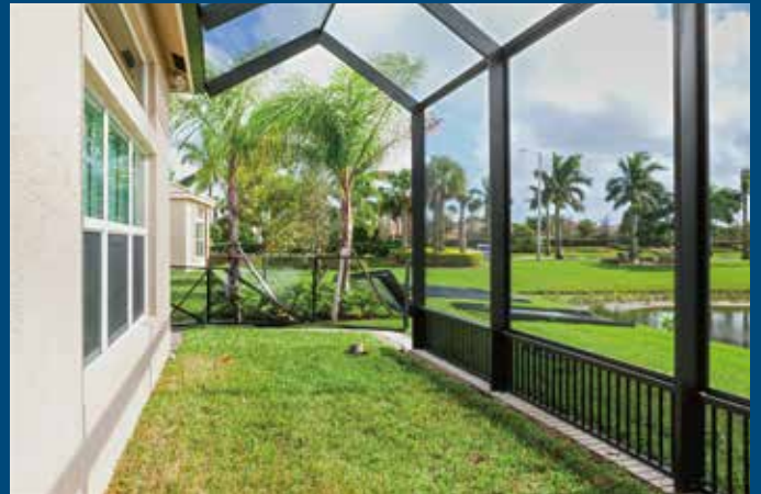
Construction Screen Installation
